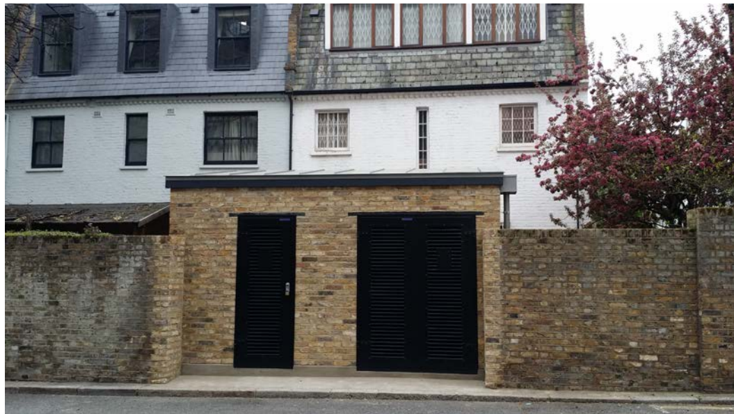
Photo to shows doors
